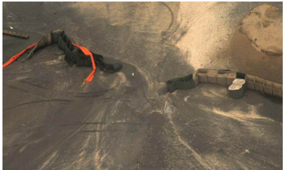
LAFOURCHE PARISH, La. – High winds and storm tides caused a breach in the Hesco baskets in East Port Fourchon Beach, La. Photo courtesy of U.S. Coast Guard
