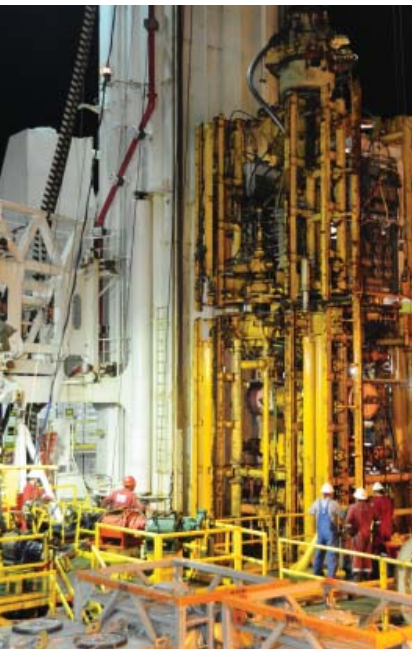
GULF OF MEXICO –The damaged blowout preventer and the lower marine riser package were removed and placed aboard the Q4000. Photo courtesy of U.S. Coast Guard
