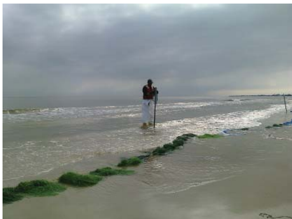
DAUPHIN ISLAND, Ala. – An oil spill worker posts stanchions to ensure that the snare booms remain along the shoreline. Photo courtesy of BP
