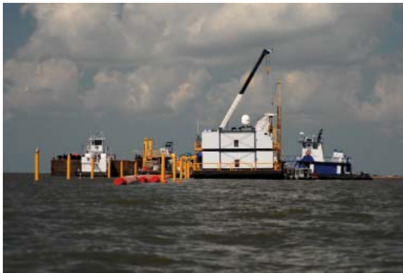
GRAND ISLE, La. – A section of rigid pipe boom, which is more resistant to rough seas, is deployed in the waters near Grand Isle to help contain oil from the Deepwater Horizon spill. Photo courtesy of U.S. Air Force
